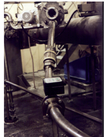
Installation monitoring and reporting the flow rate of powdered materials
